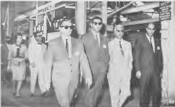
ANTILLEAN LEGISLATORS are shown above, left, during their tour of the Mechanical Shops. They emerge from the General Office Building, above right, after conferring with Lago's Board of Directors as a highlight of their visit to the refinery.
